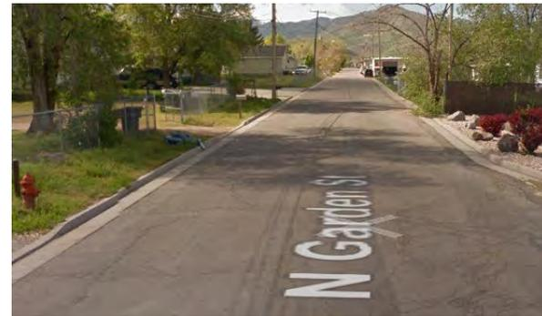
This section has curb and gutter throughout with about 26 feet of asphalt for the entire segment. With the gutter pan included the hard surface increases to 30 feet. There are 3 hydrants along this segment that are within code distances.
