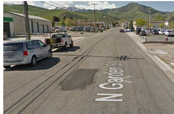
This section has asphalt widths at 30 feet throughout. There sufficient hydrants within this segment that are within code distances throughout.
