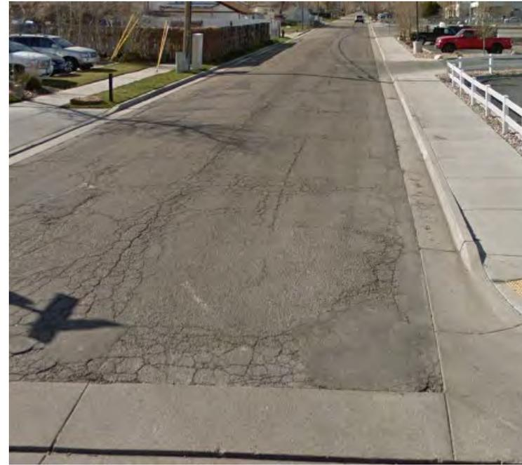
This section has about 26 feet of asphalt throughout the entire segment. The gutter pan puts the width to 30 feet of hard surface. There is sufficient coverage with fire hydrants for this section that are within code distances.
